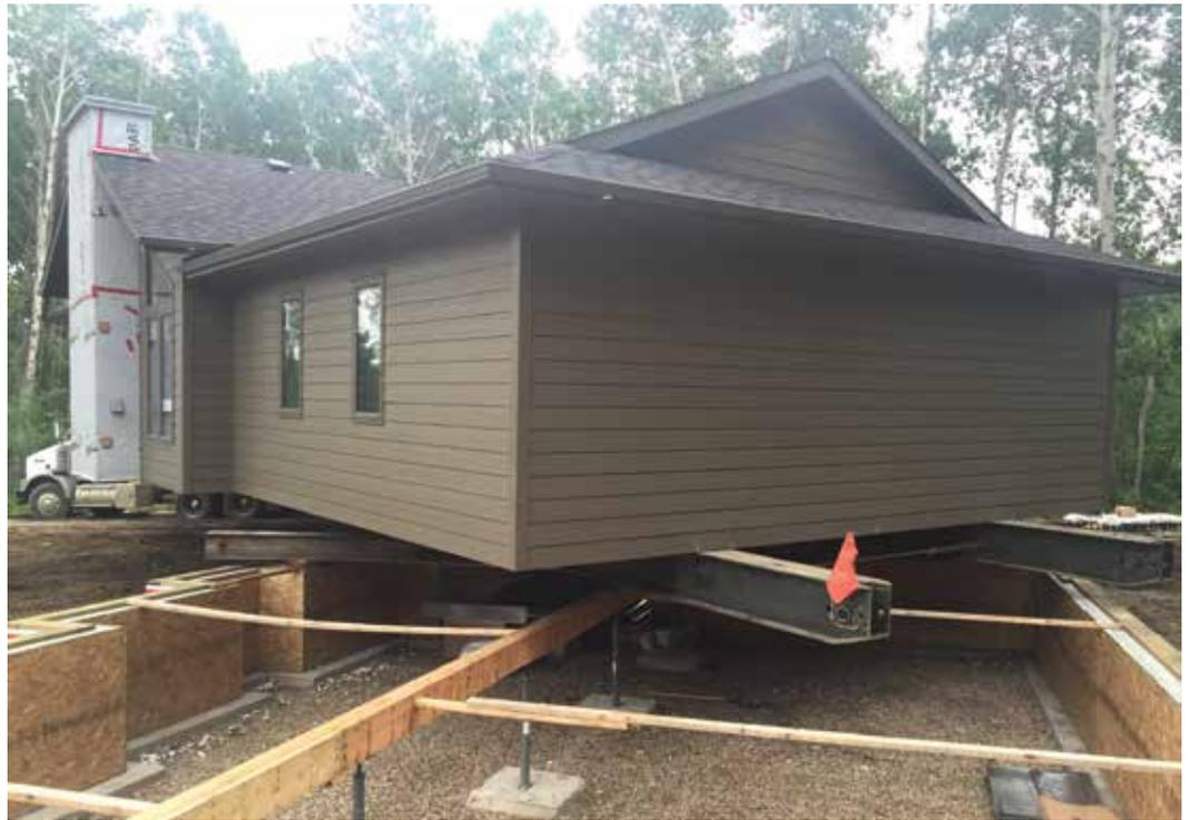
the house is placed on the foundation, care is given to make sure it is square and centered. House to Foundation joint matches the quality of on-site construction.
